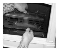
**10)** Remove all 6 screws holding the burner tray assembly in place.
